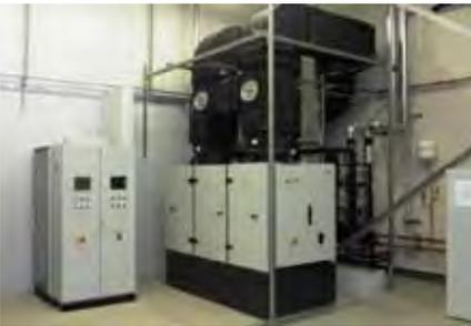
Bild 40: BHKW mit 80 kW<sub>th</sub> / 40 kVA
